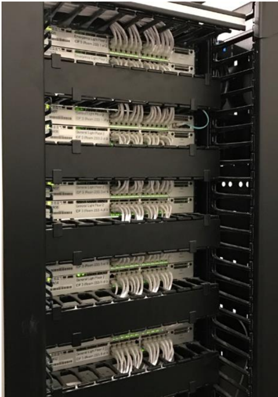
Centralized POE deployment must address NEC 726 Cable Heat Rise
